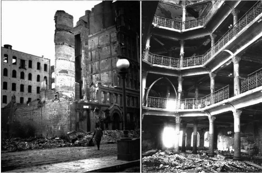
FIGURE 27. The California Academy of Sciences following the earthquake and fire, 18 April 1906. (left) Little remains of the front Market Street building; the white building on the left is all that remains of the Academy’s museum. (right) The burned out interior of the Academy’s museum building.
